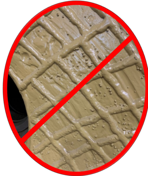
Figure 2 – Incorrect pattern on base plate
