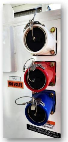
When the cables are installed into the receptacles, be sure to utilize the locking device that retains the cable within the receptacle. Between use, install the weather caps into the receptacles to protect the connections from wear.
